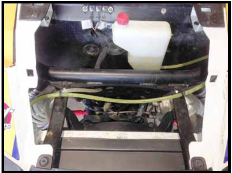
“Figure 11” Contactor Location (located under the hood)
